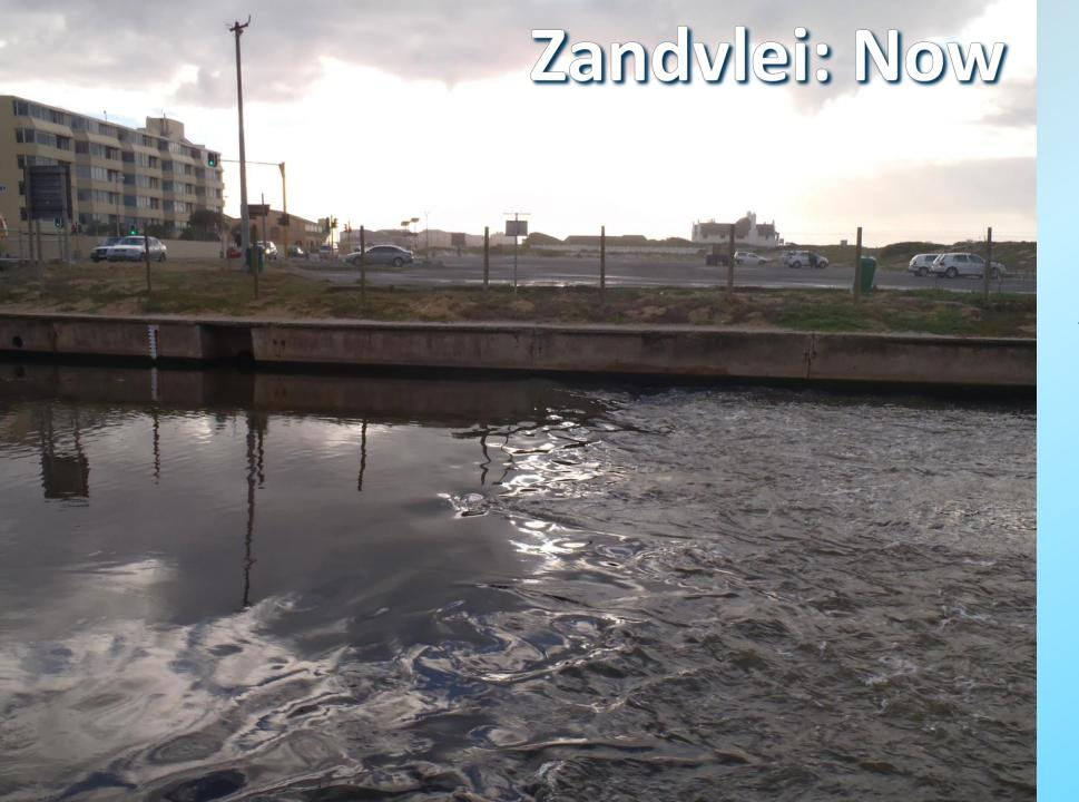
The Weir on the ebb tide: Mostly laminar flow above and turbulent flow below
